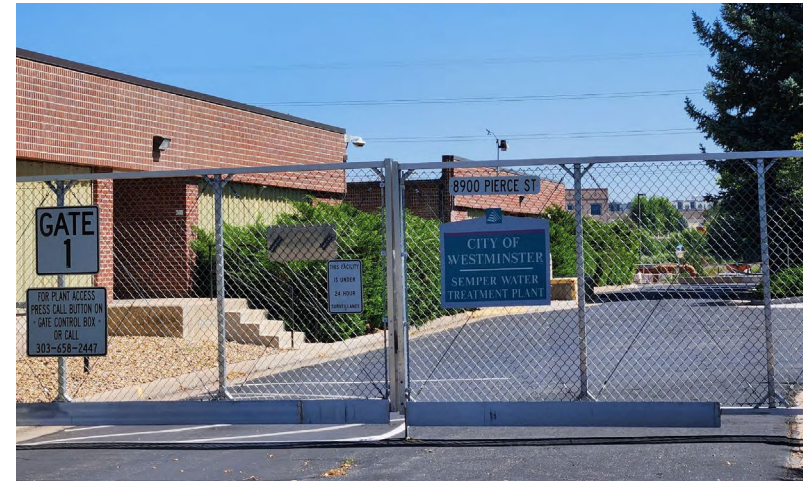
Aging Semper Water Treatment Facility
