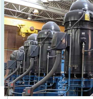
The City of Westminster is investing \$15 million to rehabilitate the High Service Pump Station which delivers 80% of the water used in Westminster. Beginning in 2019, this project will replace aging equipment and add additional backup generator capacity to increase reliability in the event of a power outage.
