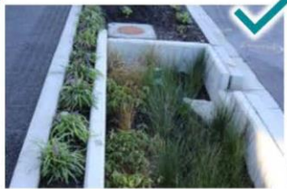
Green drainage elements
