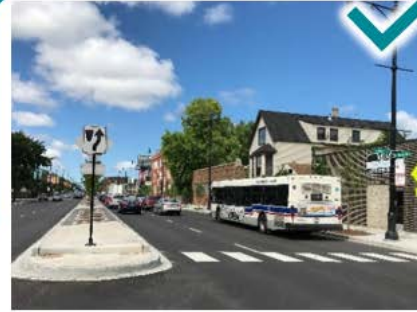
Brick or hardscape median
