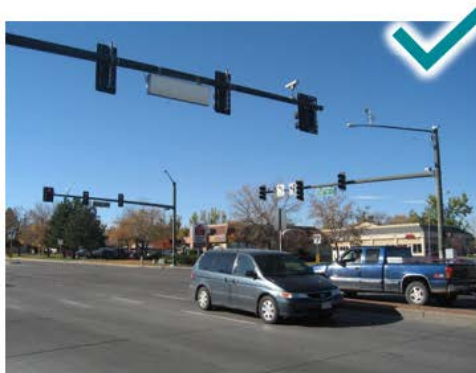
Update signal equipment - Signal Rebuilds
