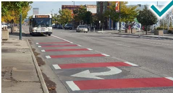
Semi-exclusive dedicated bus lanes (lanes that are reserved for buses and right turning vehicles)
