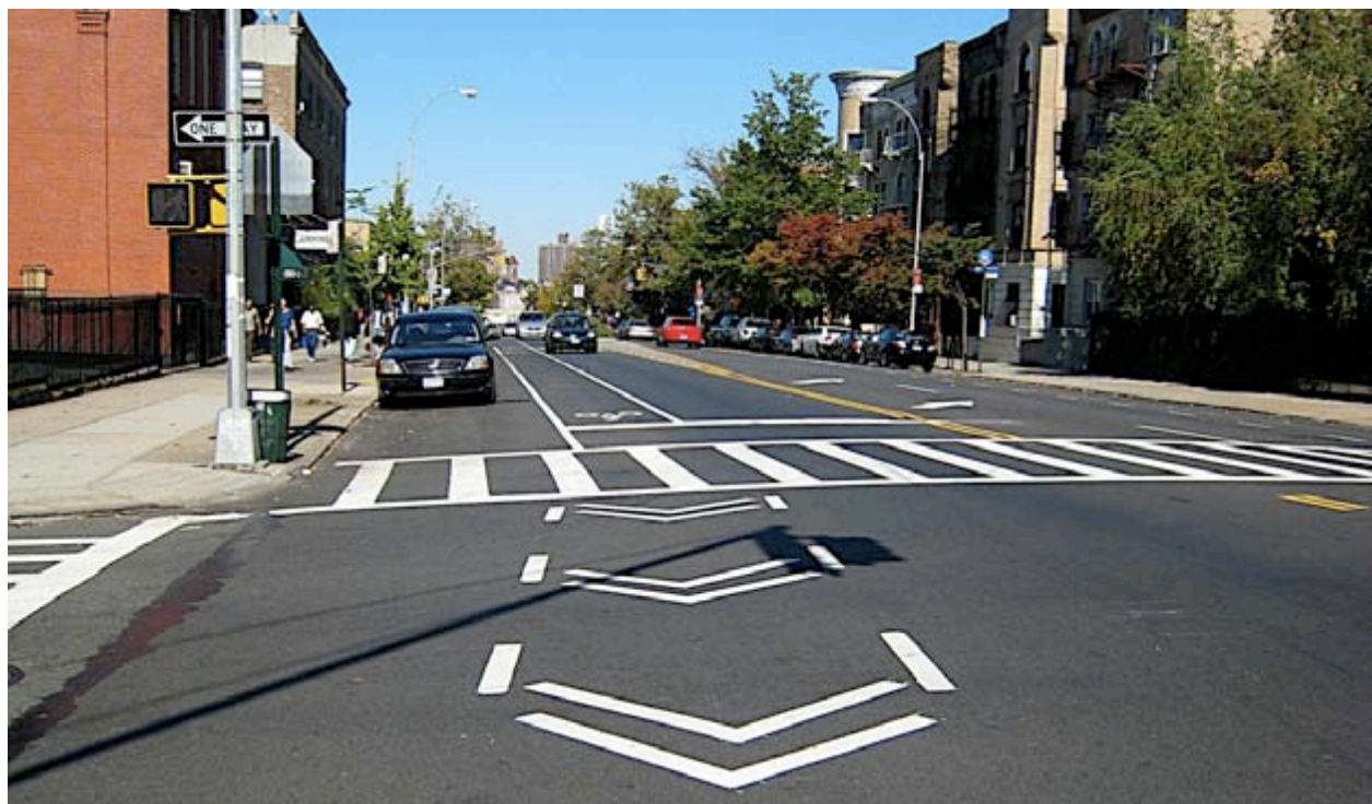
Peg-a-Tracking helps identify the proper positioning for people bicycling through an intersection. (Photo Credit: Bike Pittsburgh)
