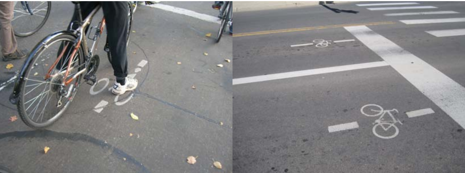
Left: This pavement marking indicates the general position where bicyclists will be detected.
