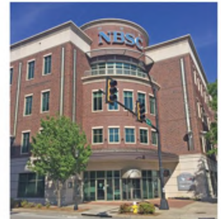
Accentuate building corners to highlight gateways, key intersections, plazas and parks through changes in massing, façade orientation and location of primary building entries.
