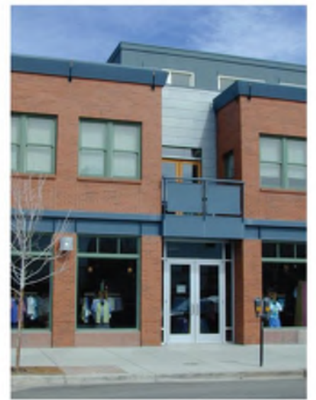
Ensure that building design is not plain and massive. Provide vertical and horizontal articulation in building mass with step-backs at upper levels and changes in materials, color and transparency, as shown above.
