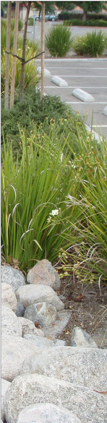
Parking Lot Bioswale
