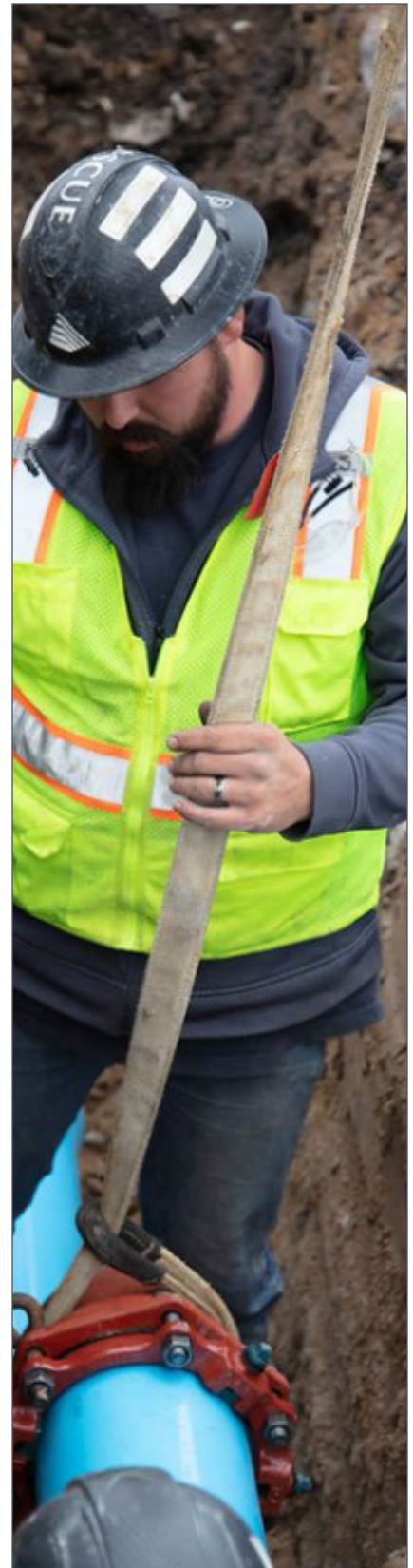
Water Main Replacement
