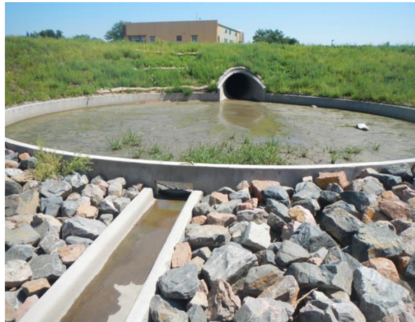
Forebay with excess sediment that needs to be removed. Vegetation growing in the forebay is a typical sign that maintenance is needed
