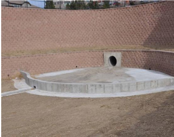
Clean forebay in working condition after recent maintenance.
