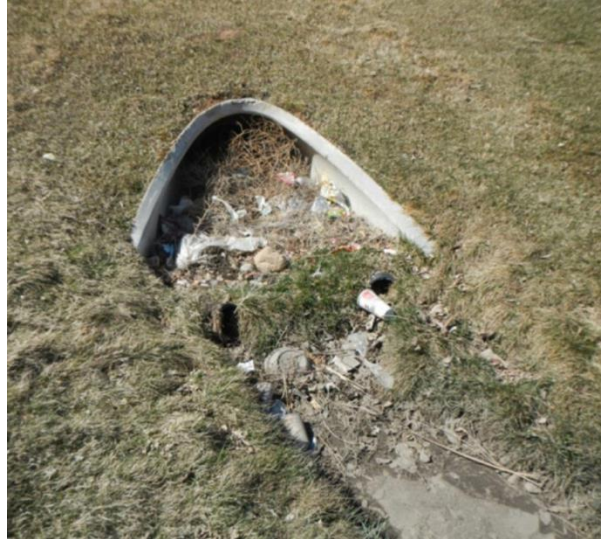
Large, woody vegetation near the outlet will eventually damage the concrete inlet pipe.
