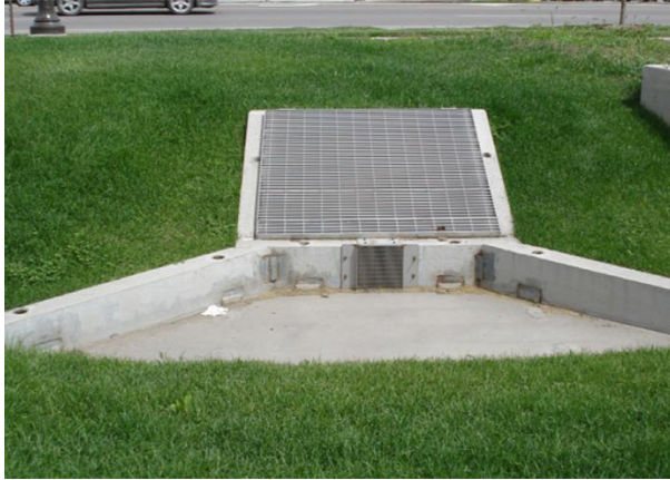
Picture of well-maintained outlet structure
