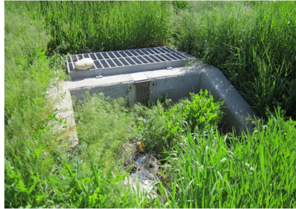
Sediment, debris and vegetation built up in front of outlet structure
