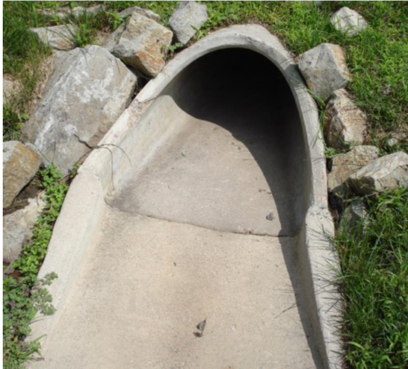
Clean inlet after proper maintenance.
