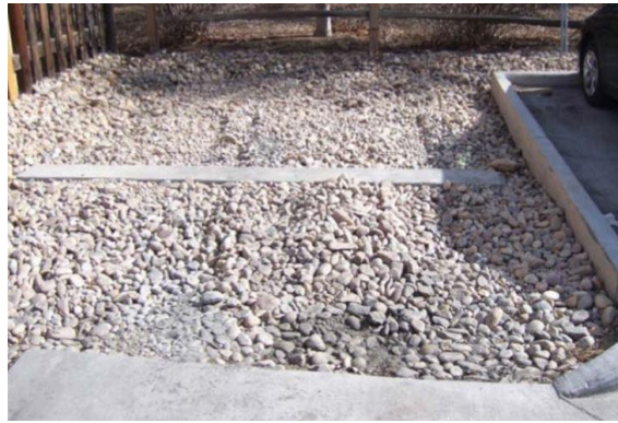
Sand filter with partial "curb" containment wall. Tracks indicate vehicles are parking/driving on top of the sand filter which can cause compaction to filter media
