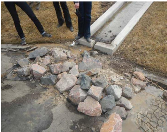
Sand filter with riprap energy dissipater. Sediment that has accumulated near the riprap should be removed periodically.
