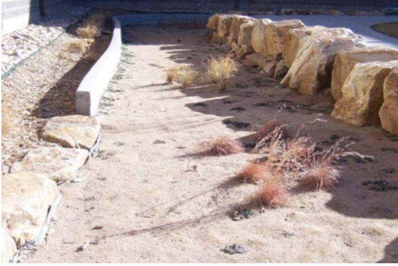
Bioretention cell with partial, concrete containment wall. Runoff will not pond to the proper design depth because the containment wall is not complete
