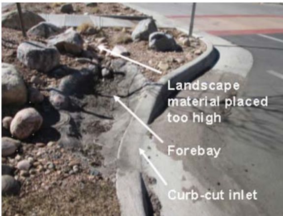
Bioretention with curb-cut inlet. Landscape material (downstream of forebay) is placed too high and runoff cannot enter the basin. Landscape material should be lowered about 3 inches below the inlet elevation
