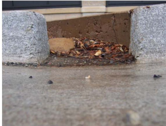
“Curb-cut” inlet with debris blocking the flow path. Landscaping material is higher than the inlet elevation, preventing flow from entering the basin. The excess landscape material near the inlet should be removed to 3 inches below the inlet.
