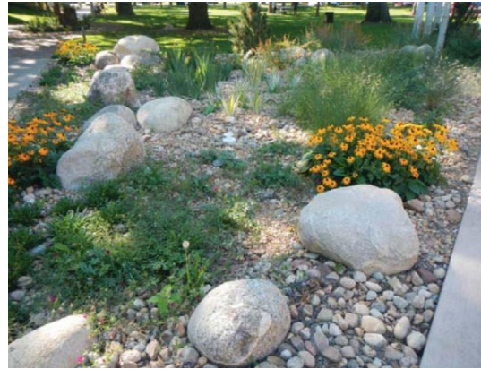
Bioretention with healthy and well-dispersed vegetation
