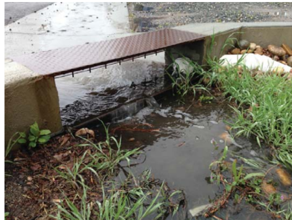
Bioretention with curb-cut inlet showing 3 inches of “fall” into basin.
