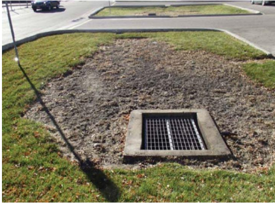
Bioretention with dead vegetation
