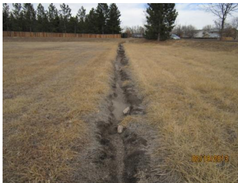
Poorly maintained BMP trickle channel
