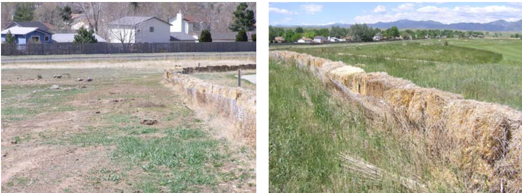
Figure 4. Photos taken in March and May 2004 (respectively) showing the straw bale and chicken wire barrier on the west side of the Westmoor prairie dog colony.
