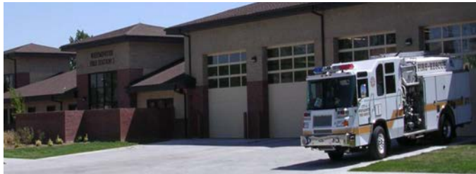
Fire Department: Firefighters and energy managers
