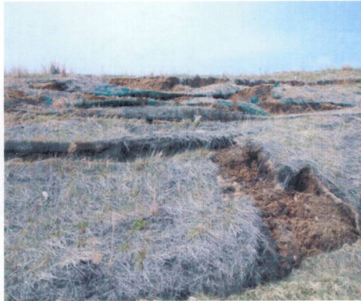
Slump below berm 7 at Original Landfill
