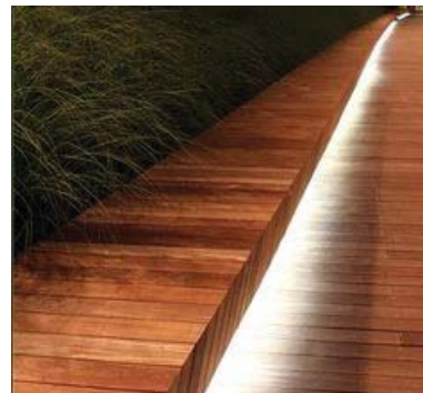
Seat-embedded strip lighting
