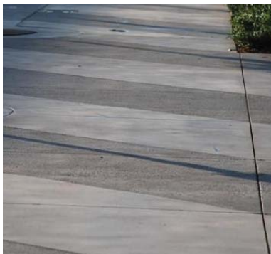
Alternating broom finish and sandblasted concrete
