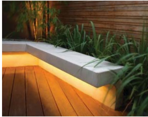
CENTRAL AVENUE - Hidden strip lighting
