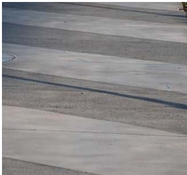
Alternate concrete finishes - 2', 4', 8' widths
