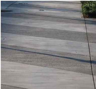
Alternating broom finish and sandblasted concrete
