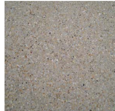
Cast concrete sidewalk
