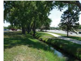
Existing Allen Ditch The historical Allen Ditch is lined with mature cottonwood trees.
