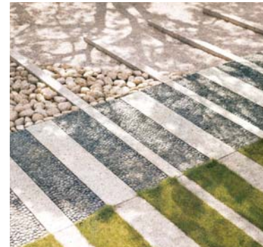
potential cut-through areas: turfstone mix set within concrete banding
