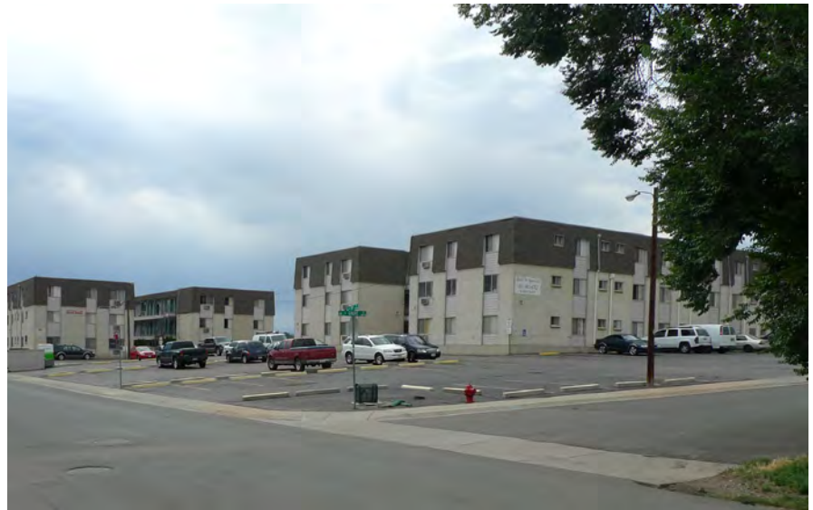
ACHA Site A view looking northwest from West 71st Avenue towards the largest parcel
