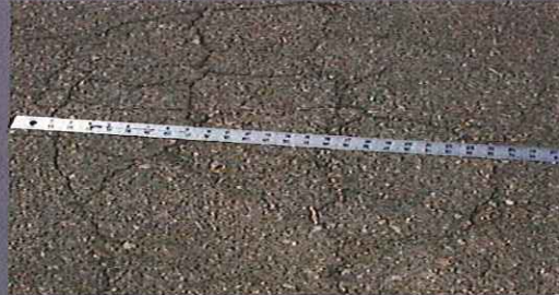
1. Alligator Cracking
