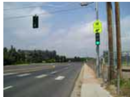
W. 88 th Ave Looking West Toward Yates
