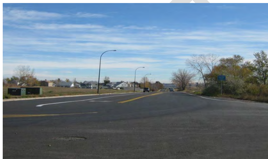
The non-standard intersection configuration and lack of pedestrian facilities at West 100 th Avenue and Simms Street creates a safety concern for pedestrians and cyclists during busy summer months
