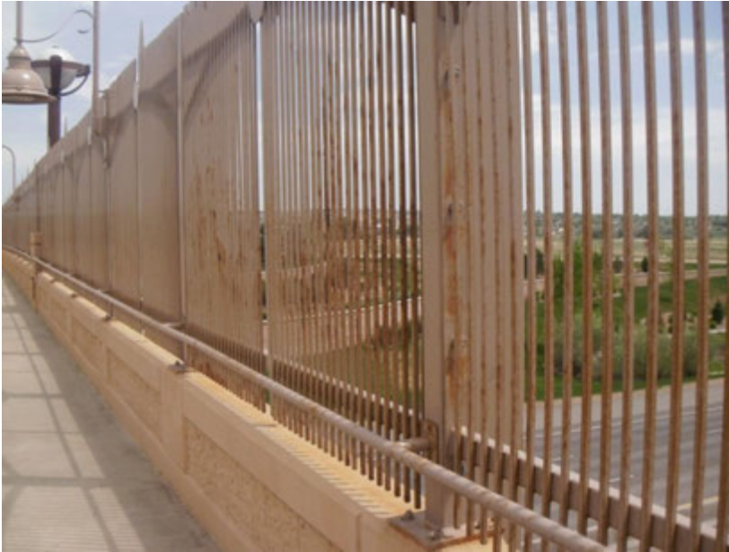
Figure 3. Overview 144th Street Bridge conditions
