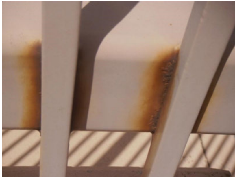
Figure 2. Overview 136th Avenue Bridge conditions
