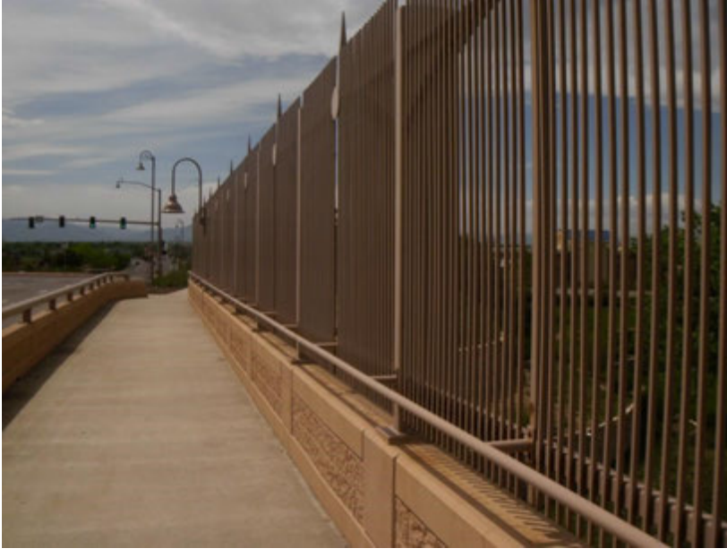
Figure 1. Overview 136th Avenue Bridge conditions
