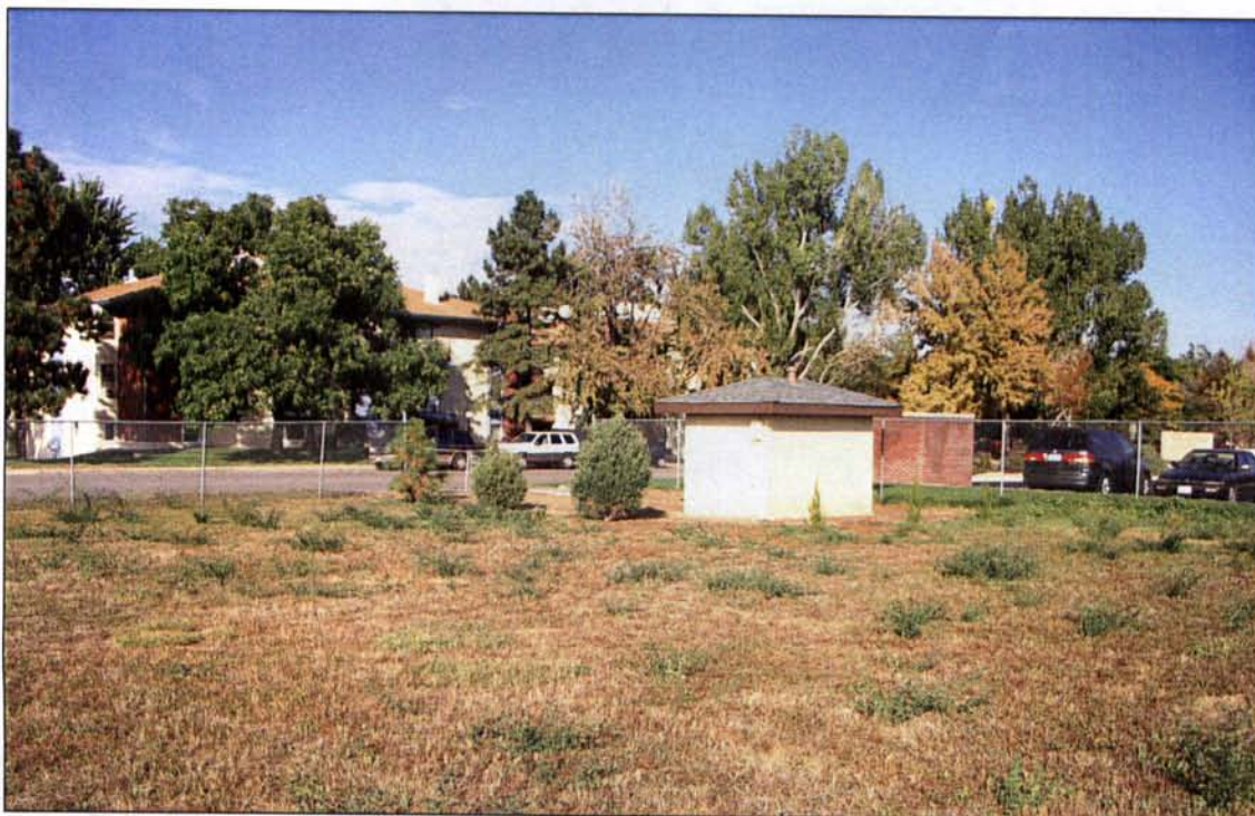
View of the gas valve house in the northeast corner of the site. View to the northeast.
