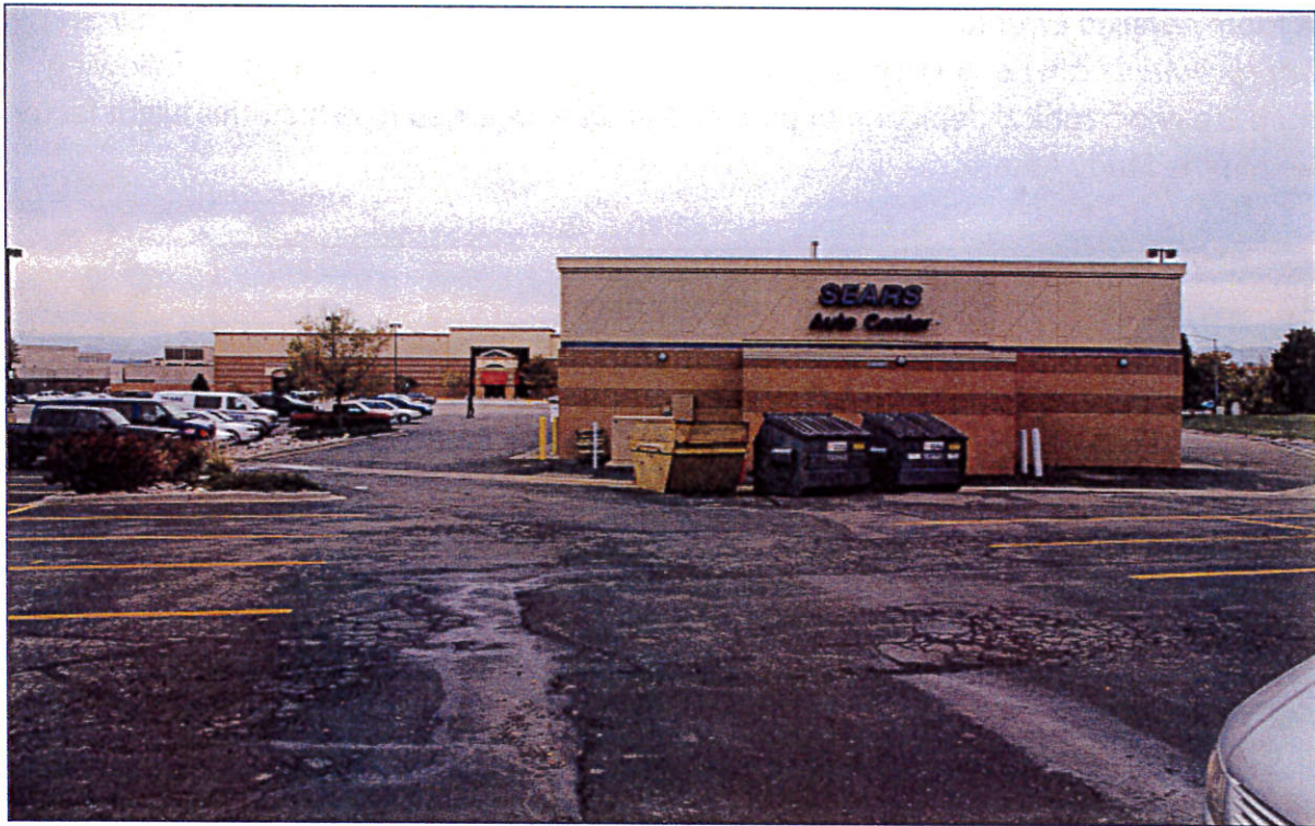
Uneven and Deteriorating Parking Surfaces
