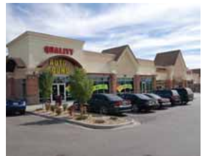
Many areas along Federal Boulevard comprise older commercial strip centers set back from the street.
