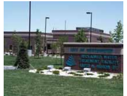
Big Dry Creek Reclaimed Plant.
