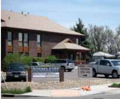
Portions of the Harris Park District reflect the city's history while other areas have opportunity for unique and complementary infill.
