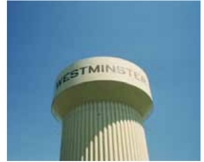
Above, the Hyrdopillar provides additional water storage for the city.
