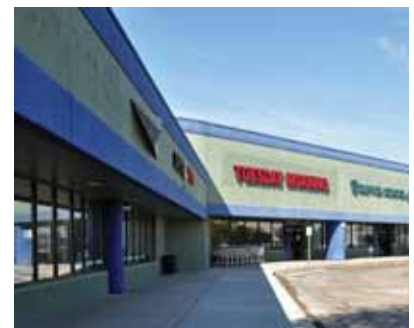
LaBelle’s Plaza, extending south from 88th Avenue on the west side of Sheridan Boulevard, is an older commercial strip center that is nearing the end of its building lifecycle.
