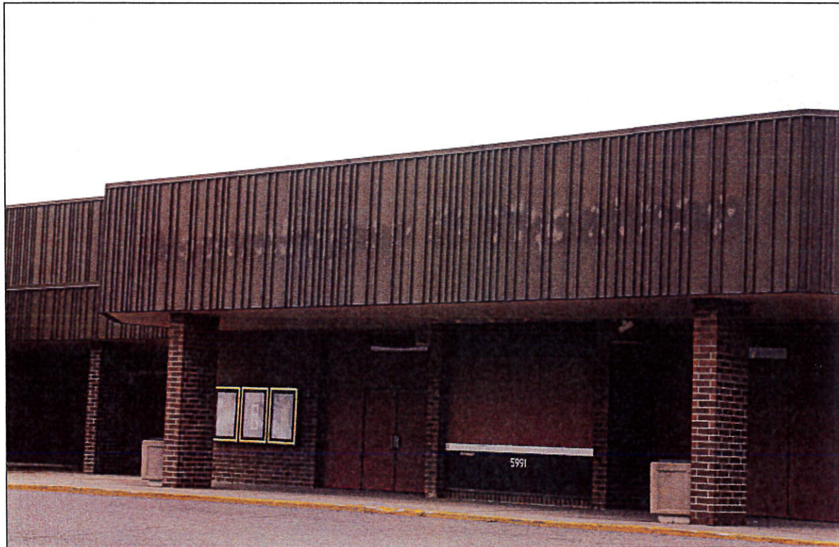
Large Exterior Retail Spaces Sit Vacant
