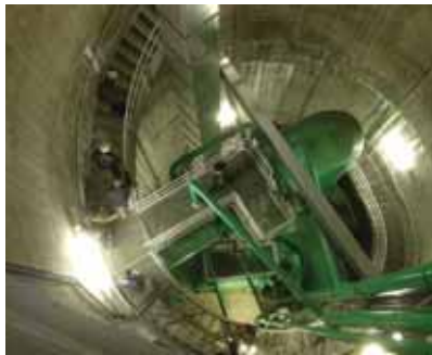
Above, Clear Creek is a source of the city's raw water supply. Below, a shaft within the Standley Lake Dam.
