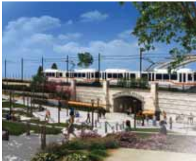
The Westminster Station, at approximately 70th Avenue and Irving Street, will open in 2016. The station and adjoining plazas parks and development will create a new transit-oriented destination and district in the city.
