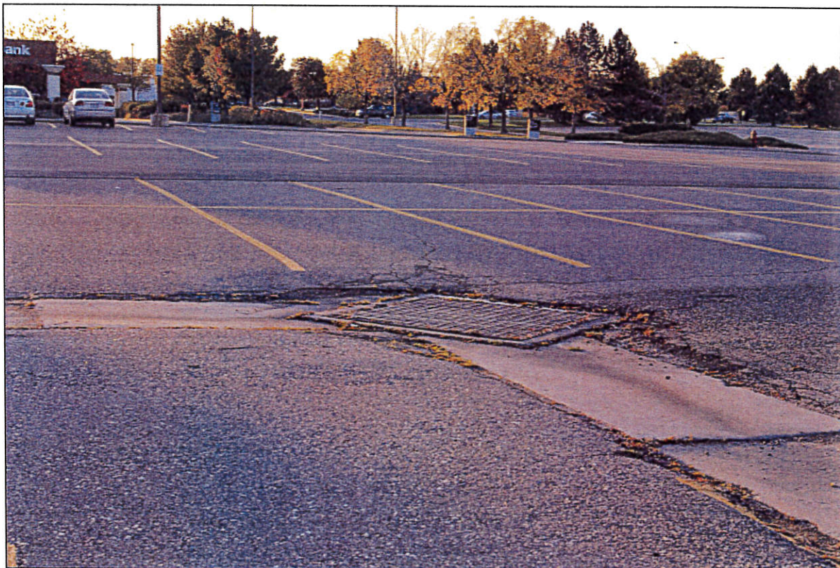
Uneven and Deteriorating Parking Surfaces
