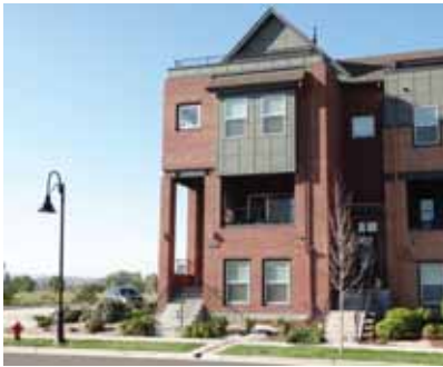
Hyland Village is a new TMUND community with development currently underway.
