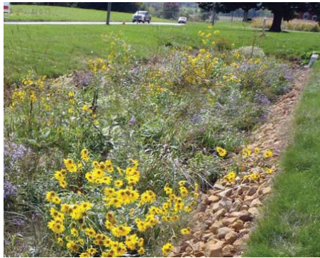
Bioswale at Park Edge
