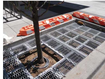
Inground Planter Under Construction
