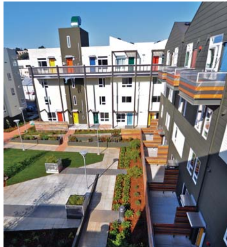
Courtyard Building Illustrative Photo
