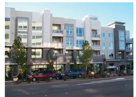
Facade Plane Breaks (4.5.1)
