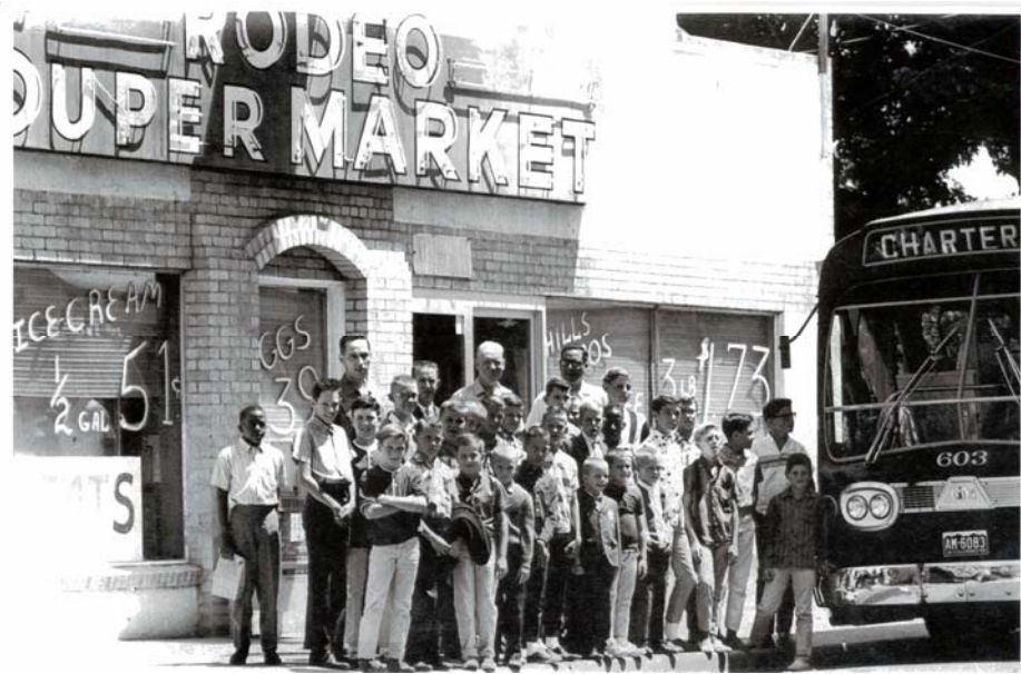
Rodeo Market Historic Façade.
