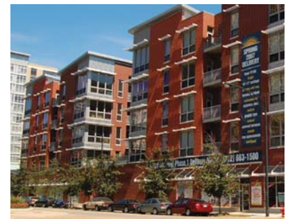
New high density residential and mixed use categories create opportunity for transit-supportive development and vibrant, mixed-use districts.
