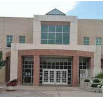
Irving Street Library, above, is the most recent addition to the city's library system. College Hill Library, below, is a shared facility with the Front Range Community College.
