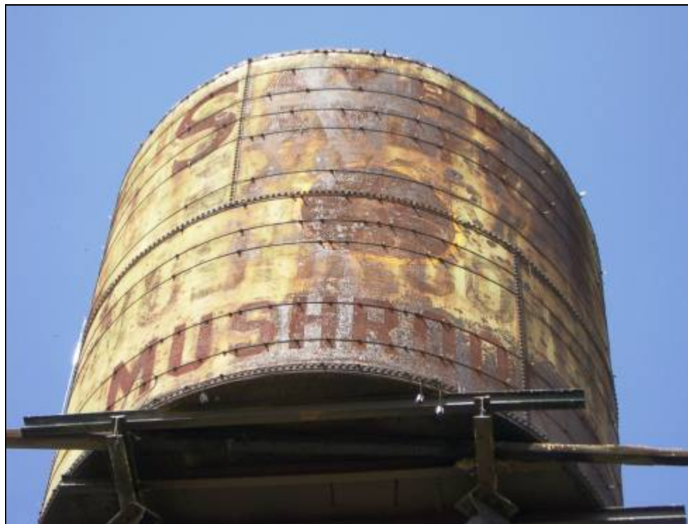
View of the water tank and its fading Savery Savory Mushrooms sign. The bands around the tank supported neon lighting.
