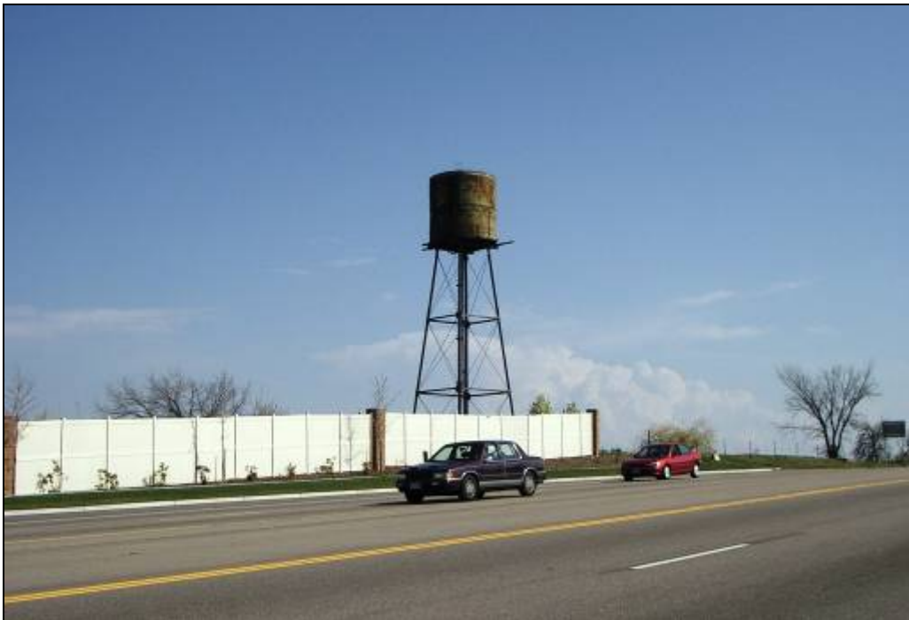
The tower from across Federal Blvd. to the northwest. View to the southeast.
