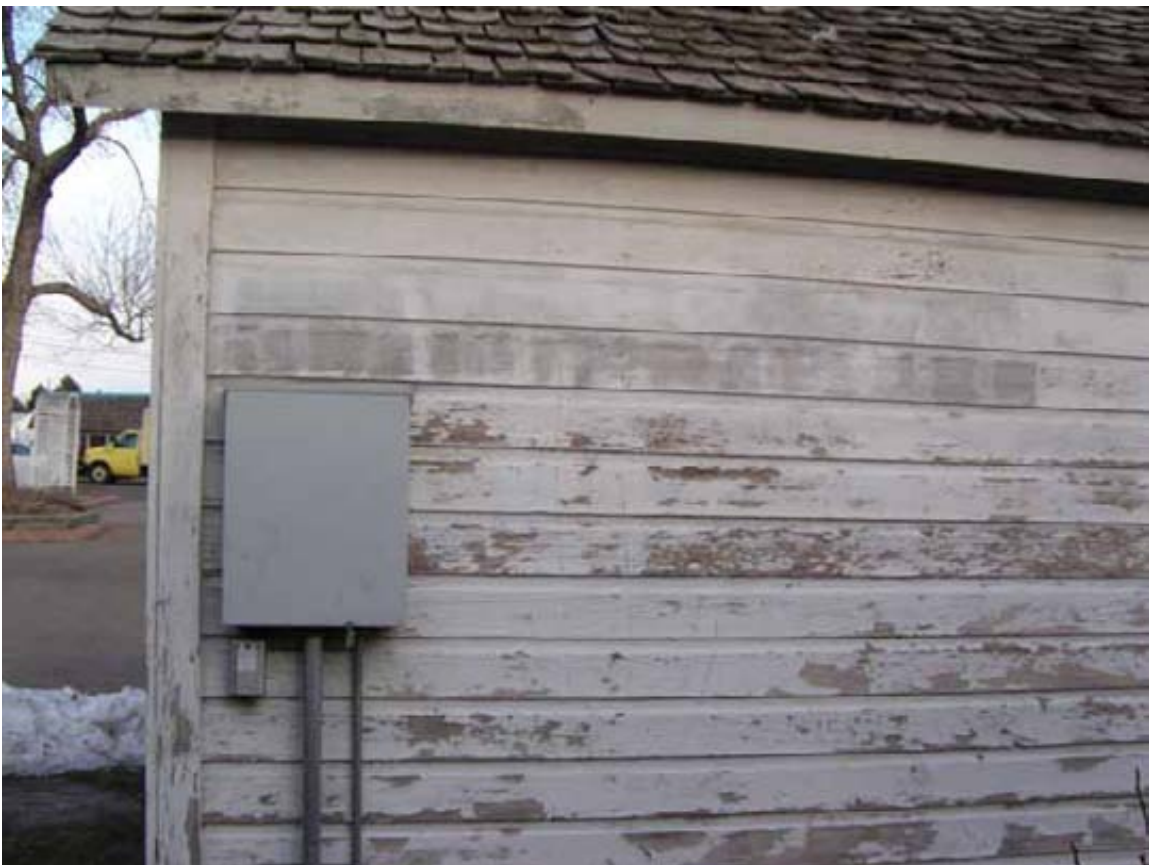
The west elevation siding is painted with sign lettering, "REAL ESTATE".
