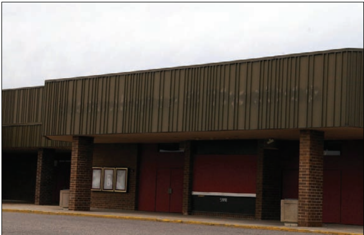
Large Exterior Retail Spaces Sit Vacant
