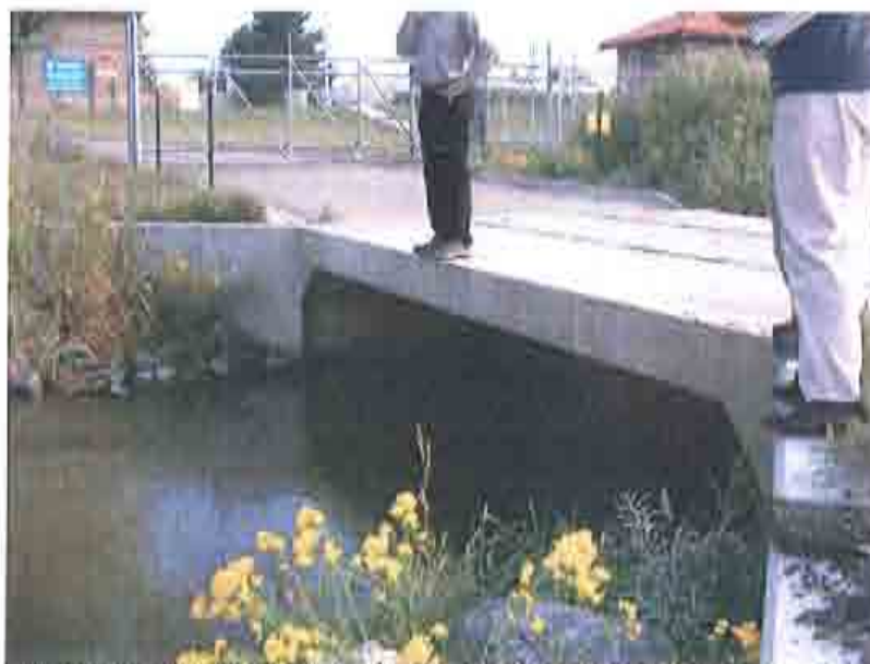
Figure 1: Westminster Big Dry Creek Wastewater Treatment Facility, Secondary Access Bridge.
