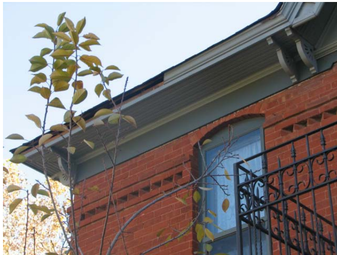
Photo shows detail of iron railing at second floor porch atop north porch.
