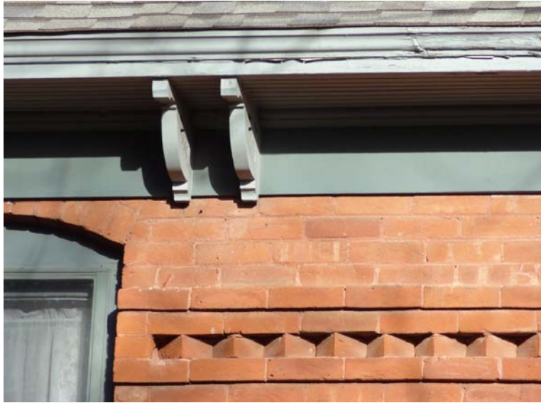
Photo shows bracket under cornice and decorative sawtooth brick courses
