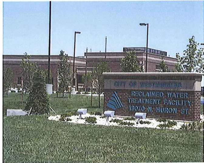
Figure 4: City of Westminster Reclaimed Water Treatment Facility
