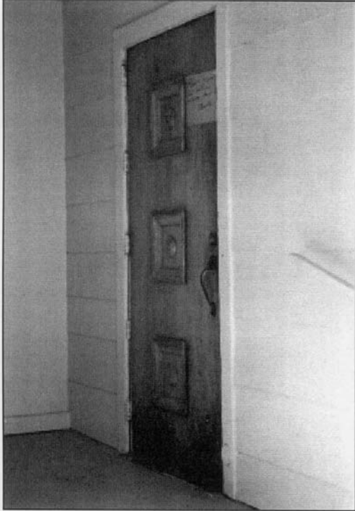
Photo No. 8: Main Entry Door
