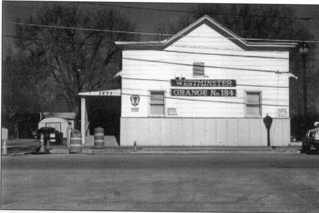
Photo No. 1: Existing South Elevation
