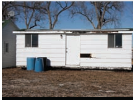
Images top to bottom: the caretaker's house, shop and garage, pump house, granary, and storage shed
