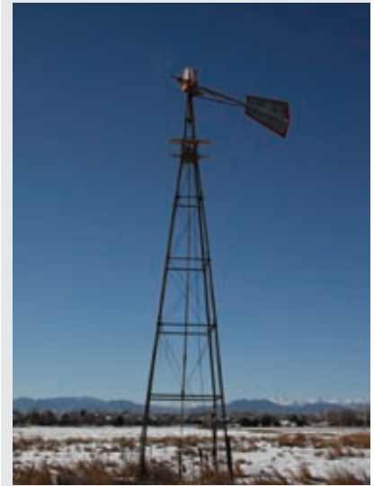
The windmill in the north pasture was used to pump water from a well into the adjacent stock tank
