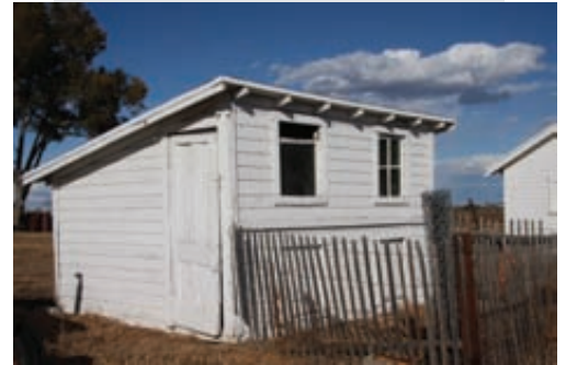
Second-level repairs would include restoring or replacing windows and doors
