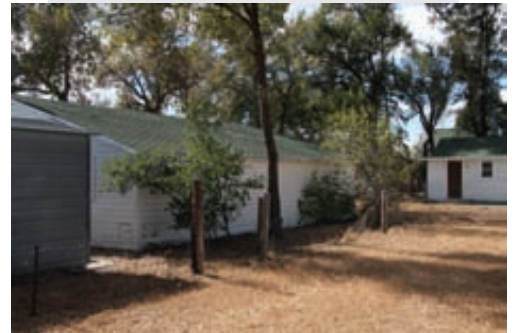
The site of former kitchen garden could be restored as part of the interpretive program
