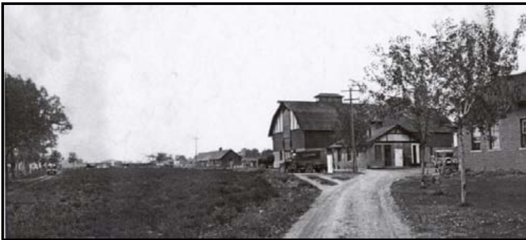
1921 Photo: Bungalow, Milk & Ice House, Dairy Barn
