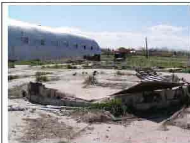
Ruins of hay feeders on concrete lot between Quonset and Dairy Barn
