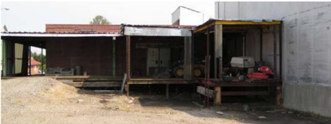
West elevation, loading dock and cooler additions
