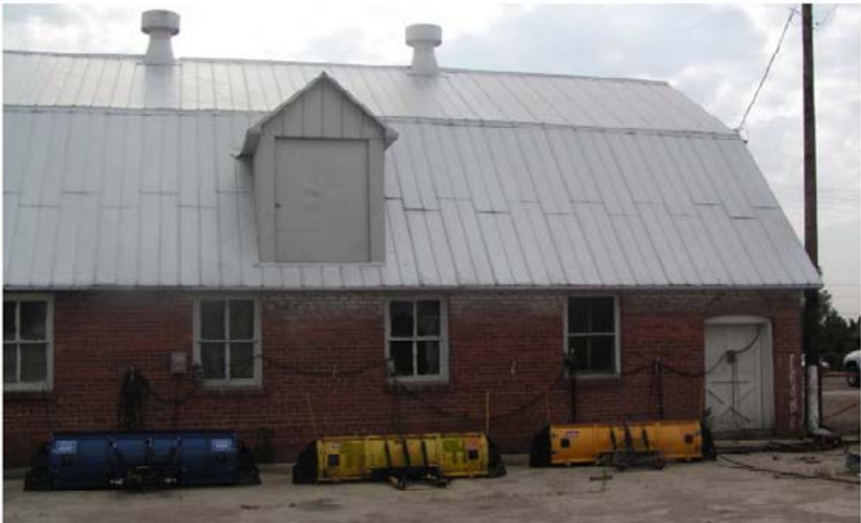
South half of west elevation
