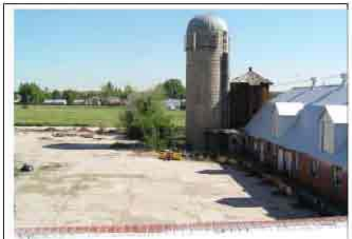
Concrete lot west of Dairy Barn
