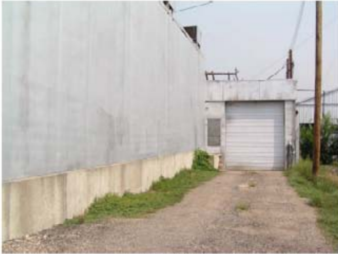
West elevation, cooler addition and west entrance to interior loading dock
