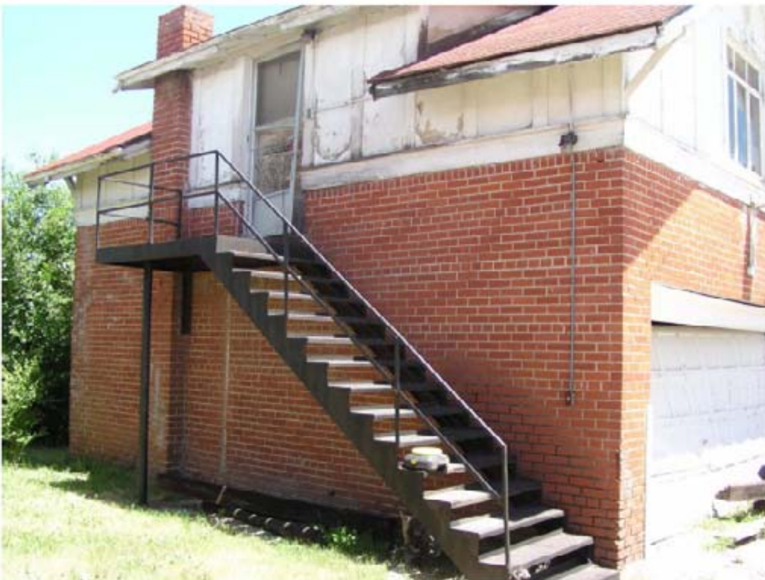
Former west elevation, relocated north elevation
