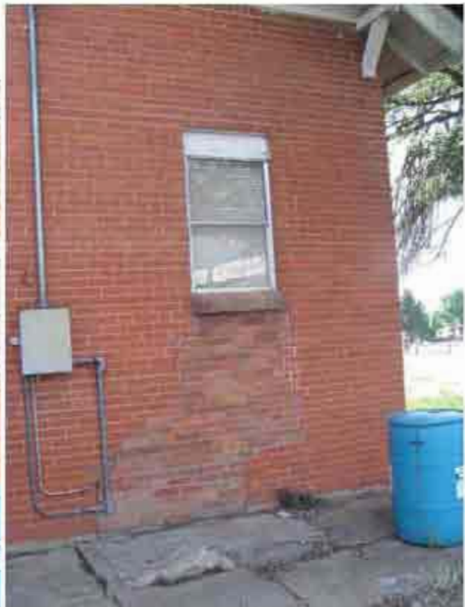
Location of original back door
