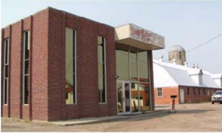
East Elevation, office addition
