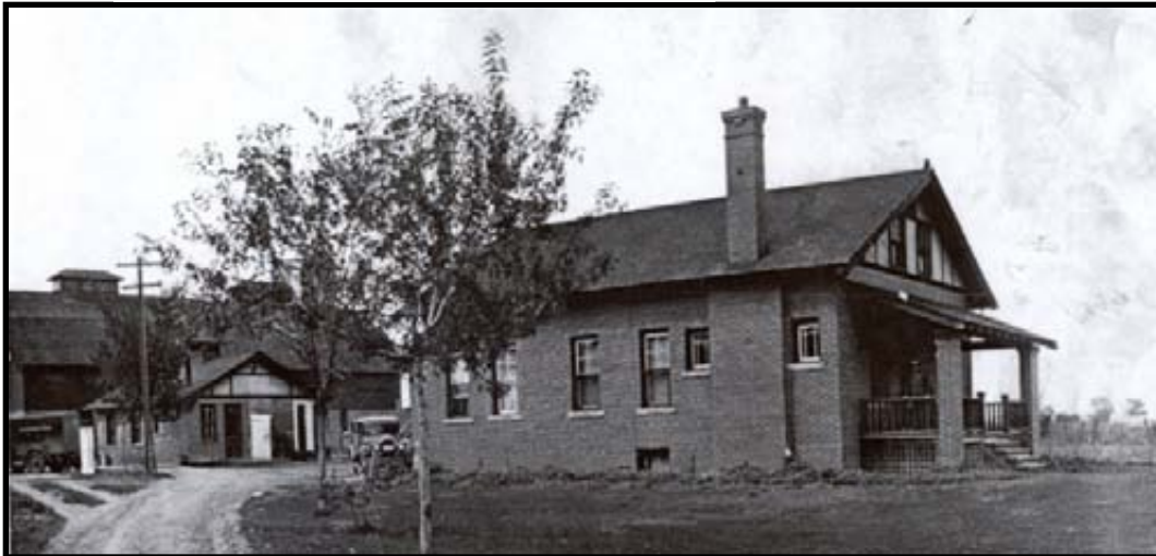
1921 Photo: Bungalow, Milk & Ice House, Dairy Barn
