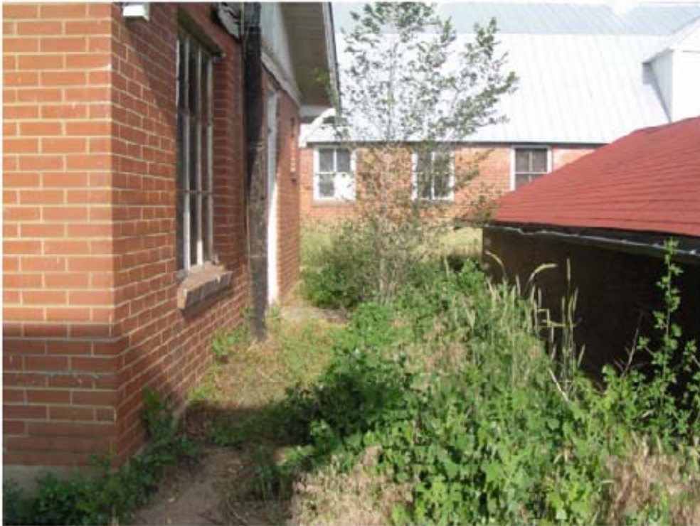
North Elevation (Pump house on right)
