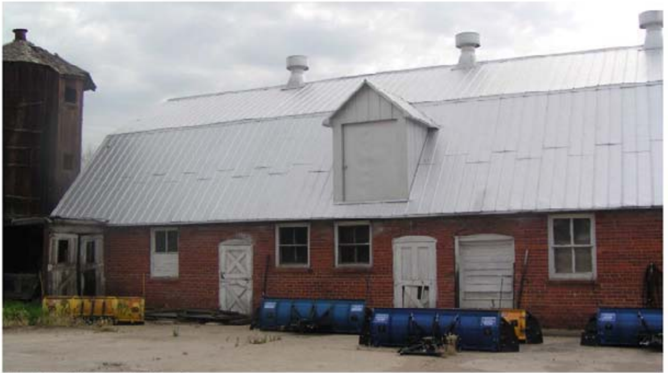
North half of west elevation
