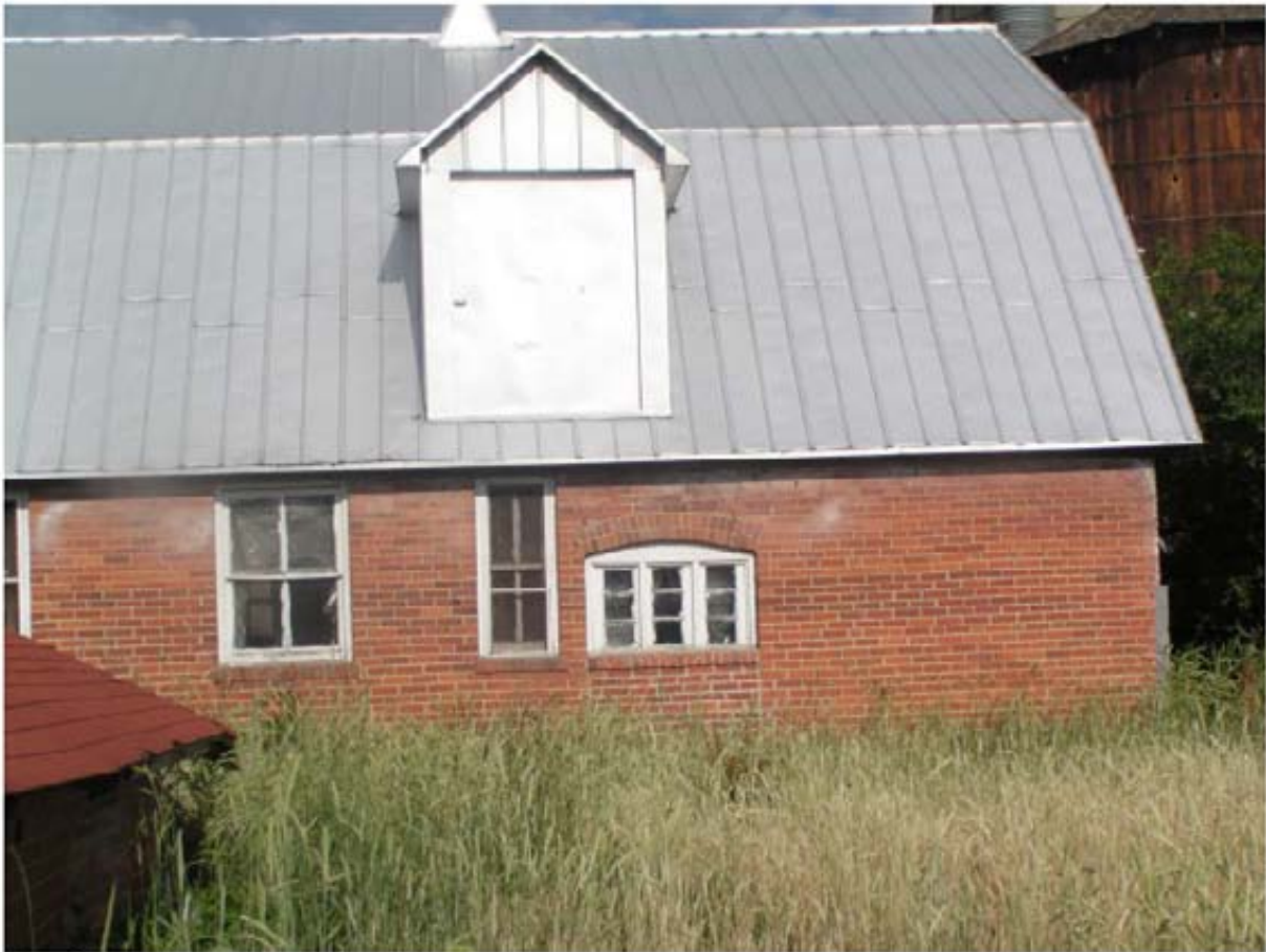
North portion of east elevation
