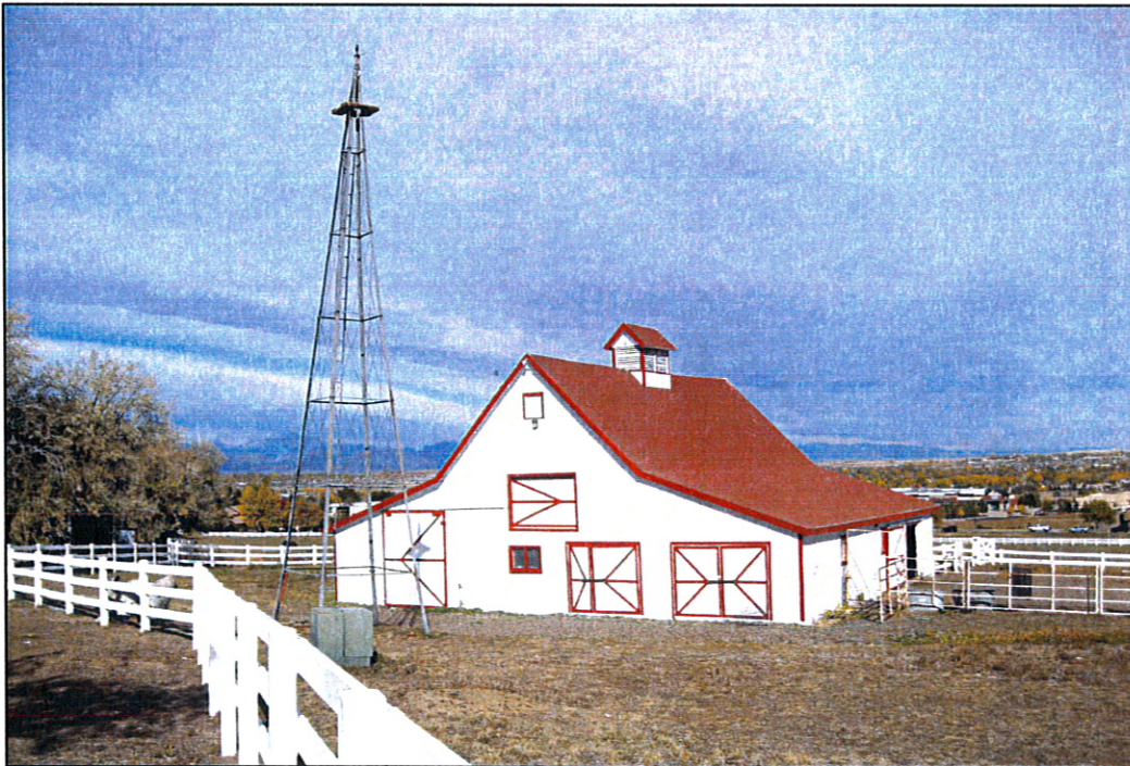
Barn & Windmill, View to the Northwest (fig. 6)
