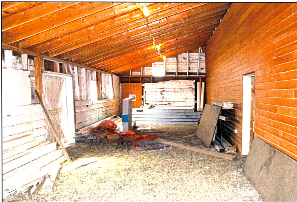
Barn Interior, West Wing (fig. 12)
