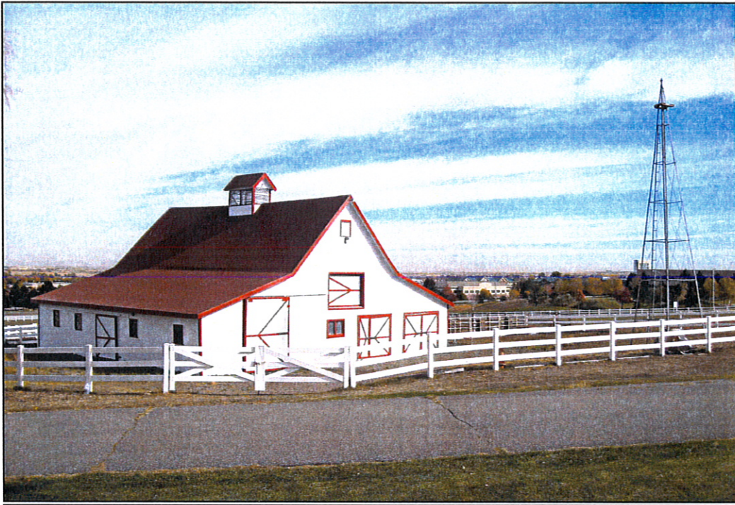
Barn & Windmill, View to the Northeast (fig. 5)
