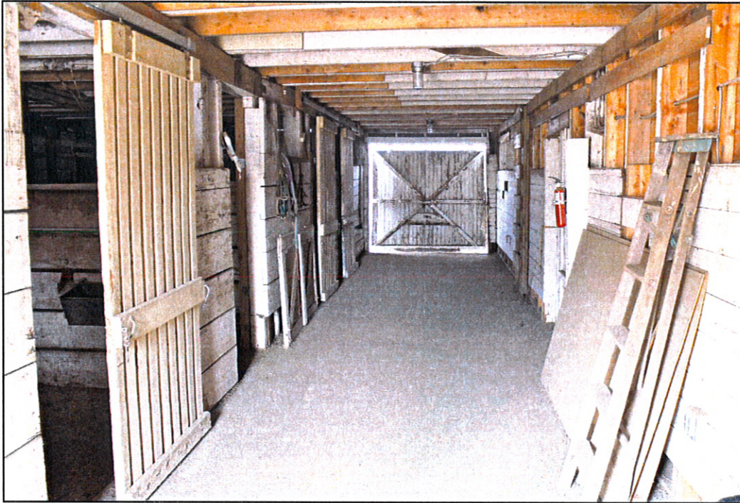
Barn Interior, Central Corridor with Horse Stalls (fig. 11)
