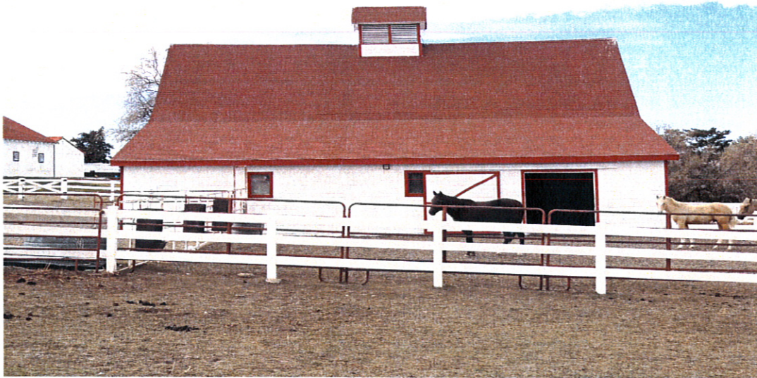
Barn, east elevation (Fig. 2)
