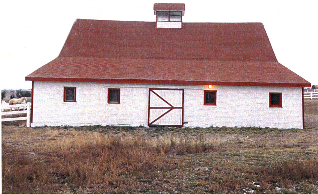
Barn, west elevation (fig. 4)
