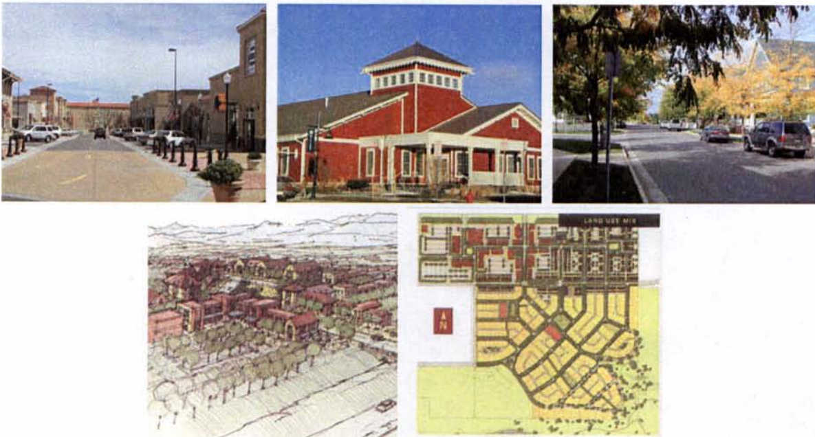
(1) Lowry Town Center mixed-use, (2) Bradburn school, (3) Single family in Longmont, (4) and (5) Bradburn, a TMUND project located in the northeast area of the City at 120 th Avenue and Lowell Boulevard, incorporates commercial, a mix of residential types, and amenities, including parks, civic uses, and a community center (Continuum, Civitas).
