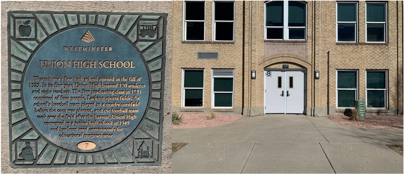
#7 3453 W 72nd Ave, walkway in front of door
