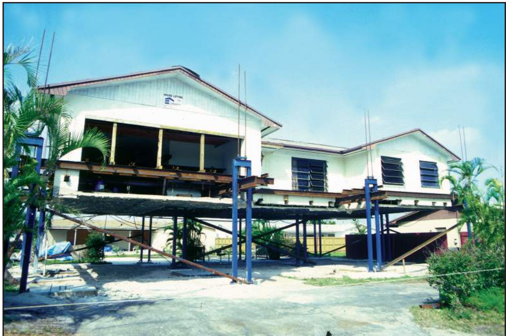
Figure 81 The house and slab were raised one full story.
