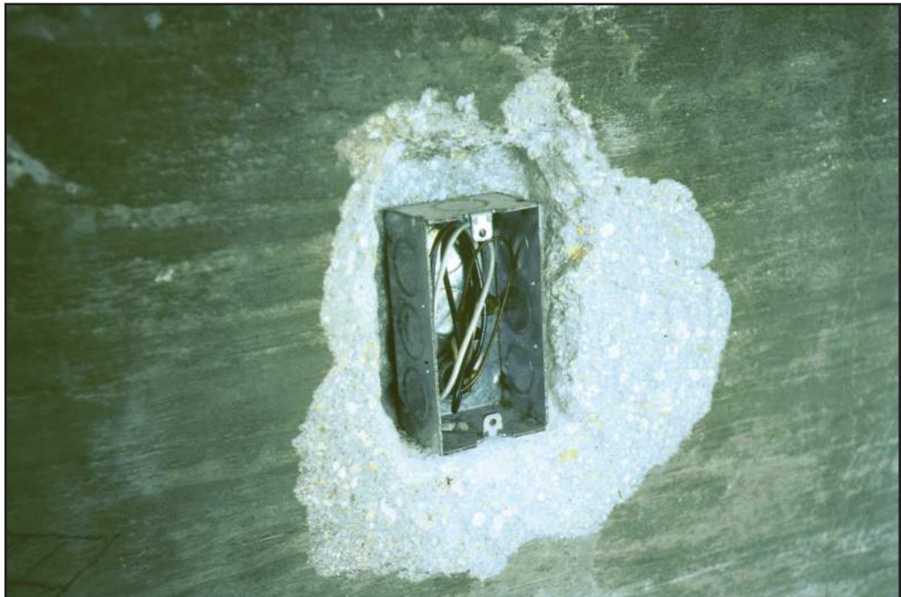
Figure 35 The electrical system is upgraded to meet current code requirements.
