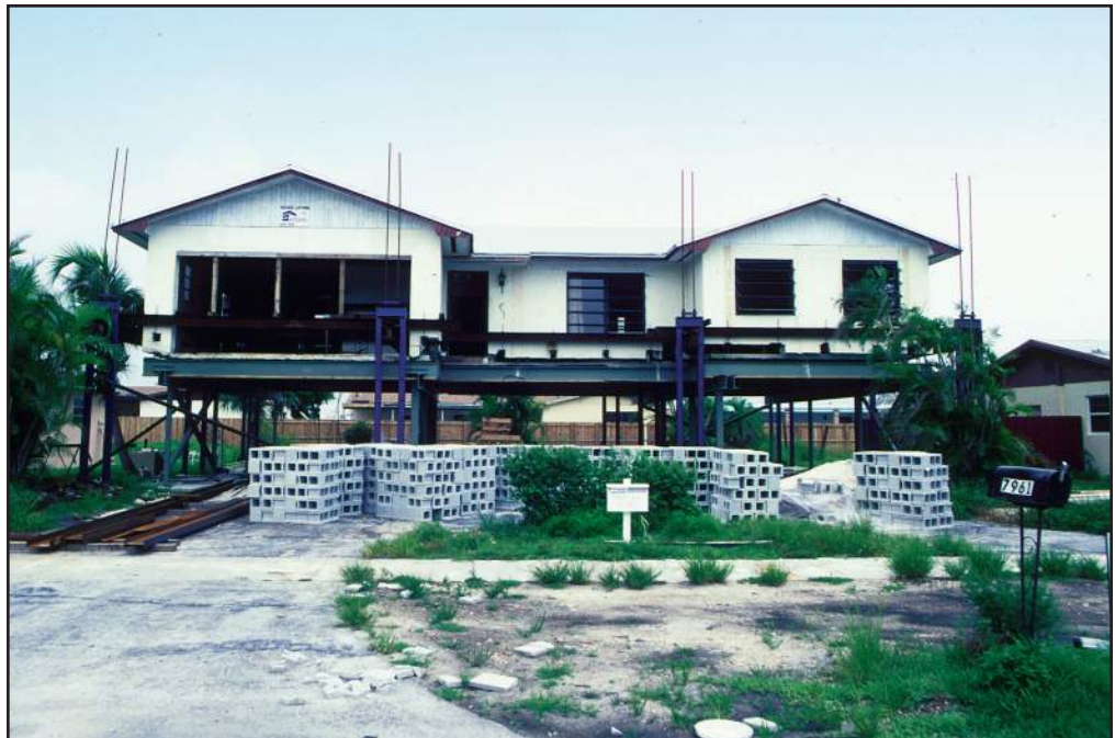
Figure 83 Concrete blocks were brought to the site ...
