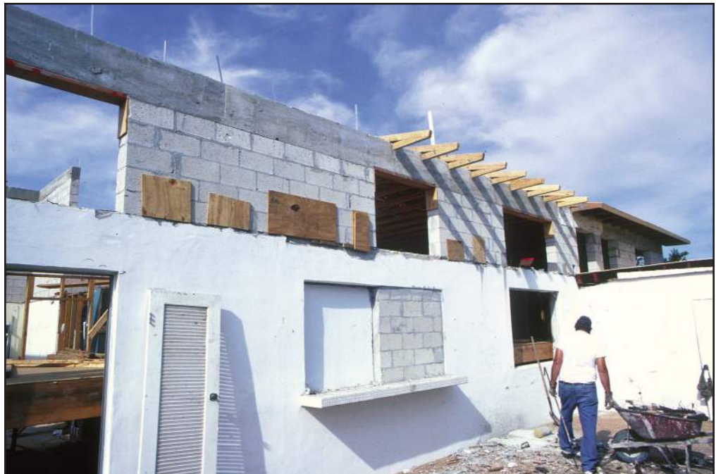
Figure 67 The extended first-story walls.
